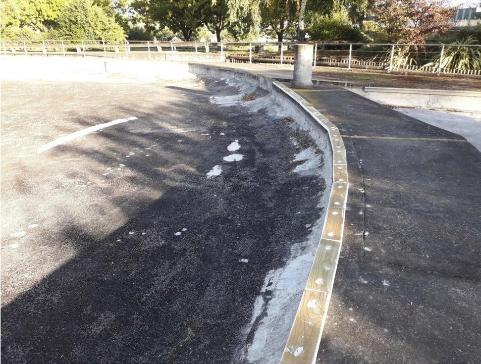
A lot of work has been done by members to get the pond ready to have a liner fitted in May. The holes in the pond have been dug out, compacted and filled, tree roots have been dealt to and the harbour area has been sealed. Wood strips have cut, painted and bolted in place around the edge of the pond for the liner to attach to. Flanges are being made to fit both the inlet and drain pipes.
