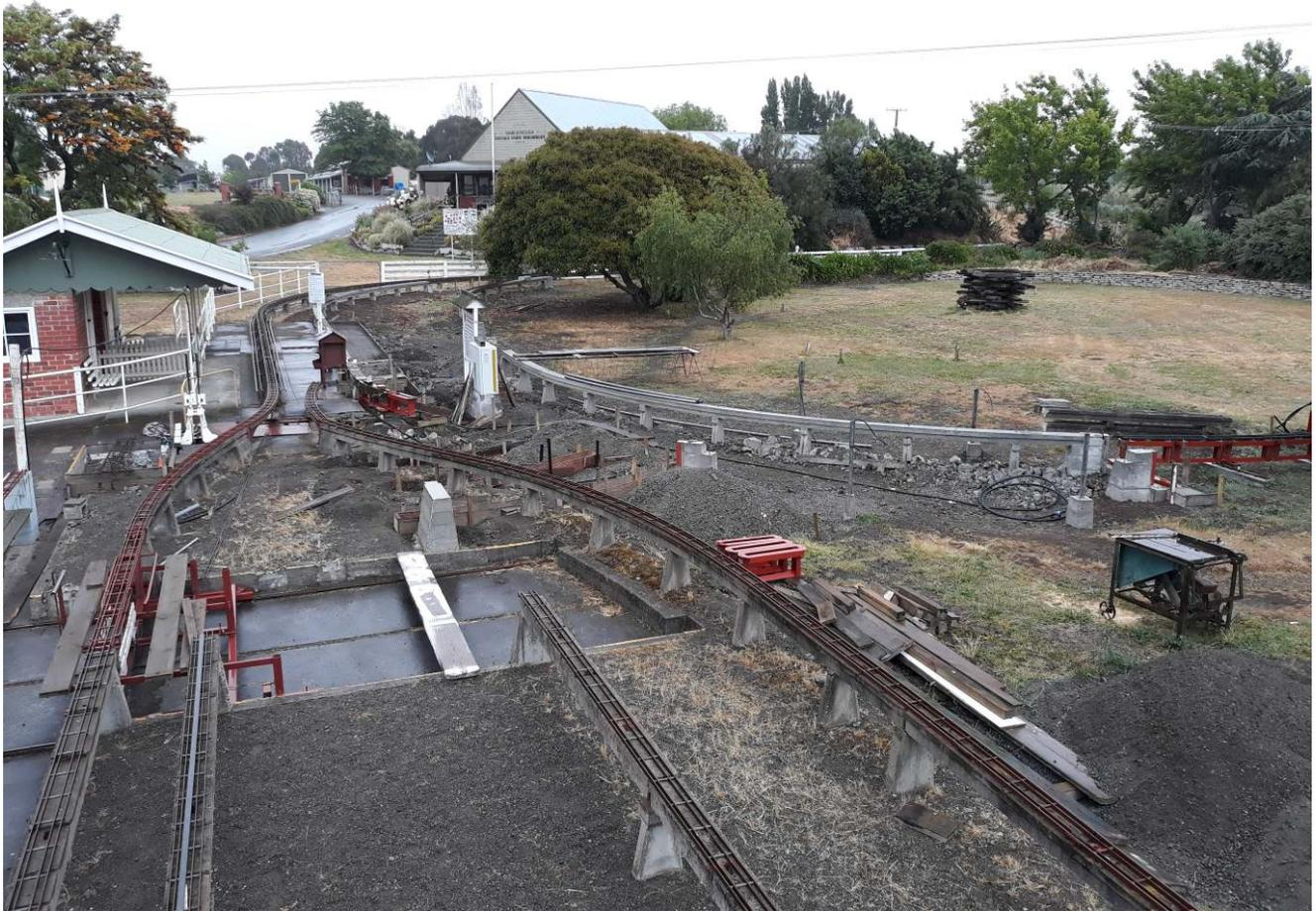
Construction of the repositioned pillars and concrete beams for the raised track and the new bypass track started early this year and is almost ready for connection to the current rail system. Mean time work on the raised track points is continuing, and replacement concrete floor and fencing in the station are underway
