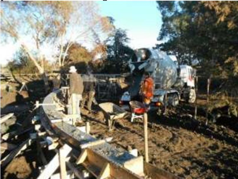
The raised track extension project continues with good progress being made but more hard fill is now required. Pouring of the last concrete piles was completed on Monday afternoon because of rain forecast. Sleepers for the tracks were cut to length and these, together with rail steel strips are to be painted before welding in-situ. WattyI etch primer is considered most suitable. Ron Perkinson to
