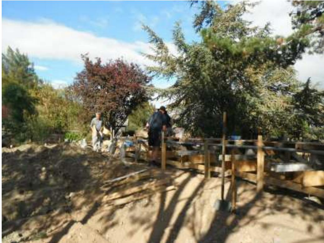
The raised track extension project is making good progress with piles of hard fill being spread around to form embankments. The curved beam sections at the north end have been poured and boxing is being set up at the south end above the tunnel.
