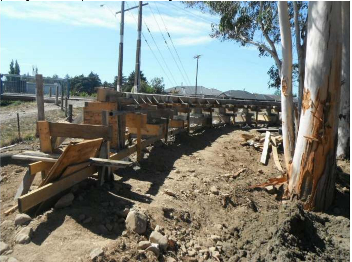
The curved sections of the track beams at the north end of the track have been poured and attention is now turning to the south curved beam sections. We have
